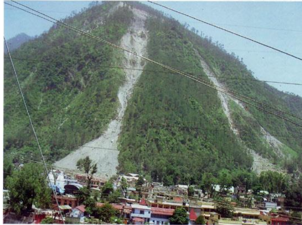
3c. Houses near landslide prone area
