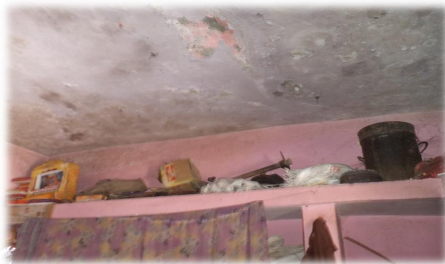
3e. Damped roof of the house
